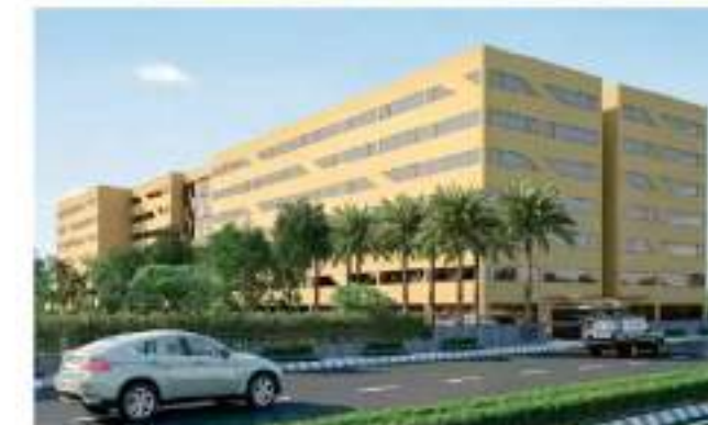
Indraprasth Business Park (Corporate Offices)
